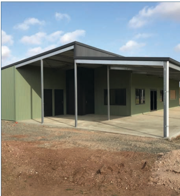
Wasleys Recreation Park clubrooms, changerooms and toilet facilities
