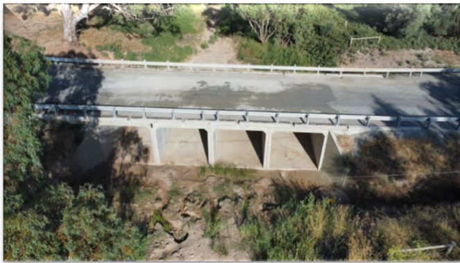
Award winning Gerald Roberts Road bridge constructed in 2021
