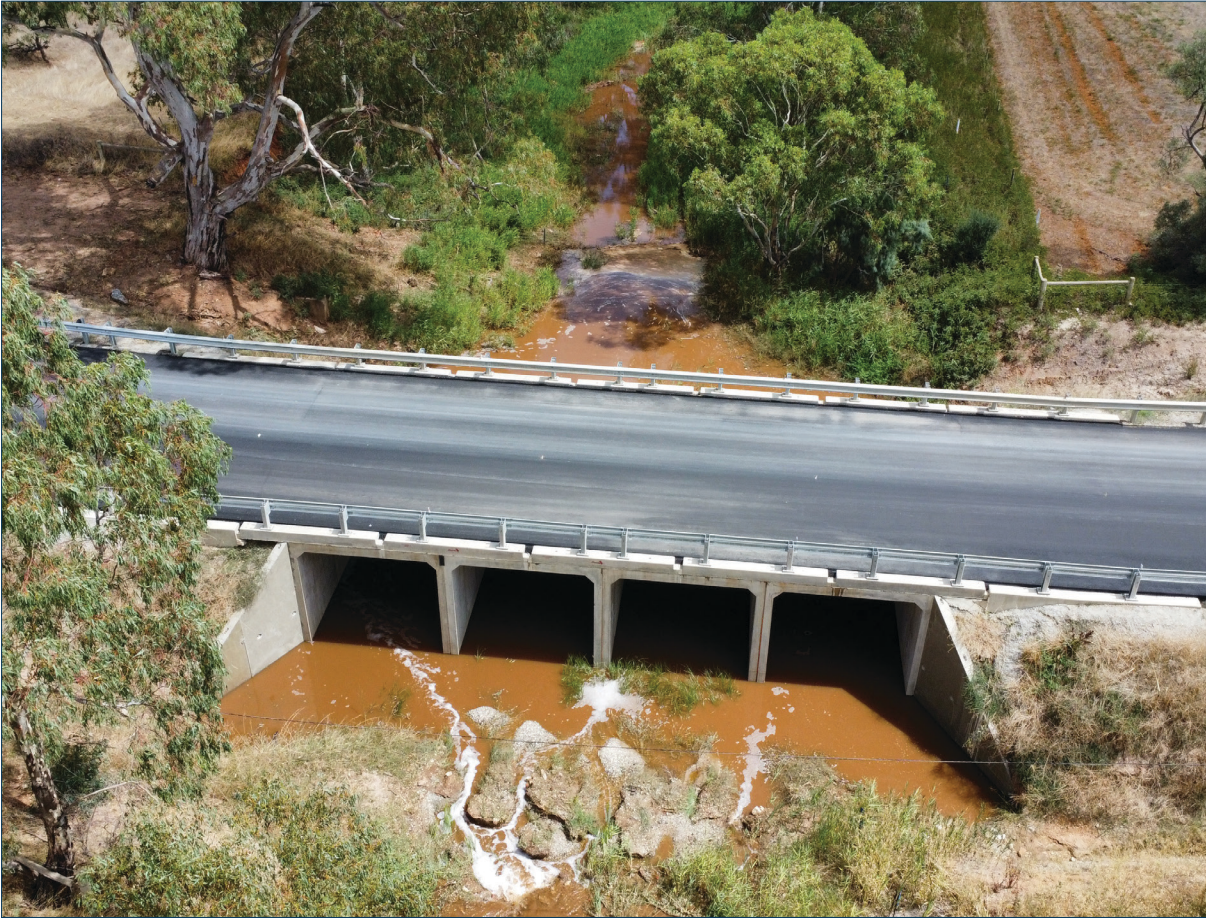
Gerald Roberts Road Bridge
