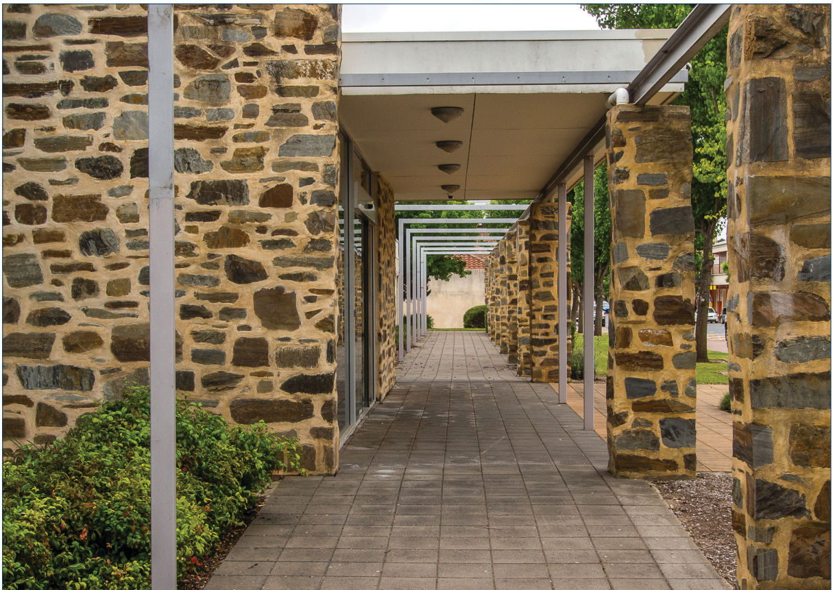
Light Regional Council Principal Office, Main Street, Kapunda
