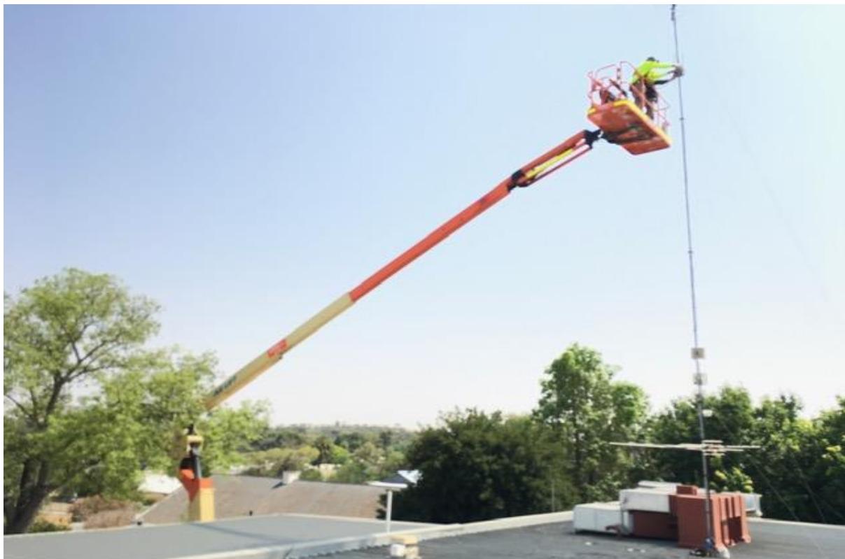
LoRaWAN antenna being installed at Main Council office at Kapunda by Damacon Services Pty Ltd
